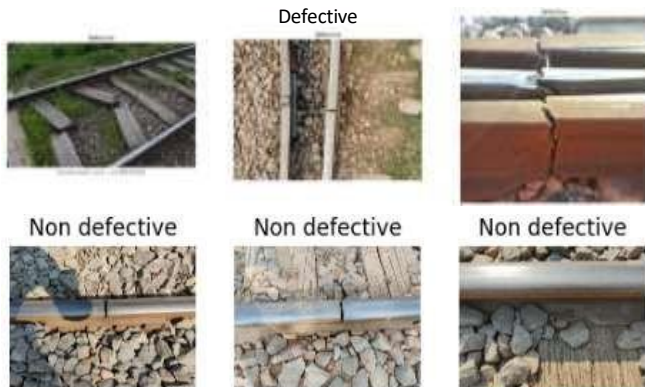
Figure 3. Sample Images of Defective and Non-Defective Railway Tracks
